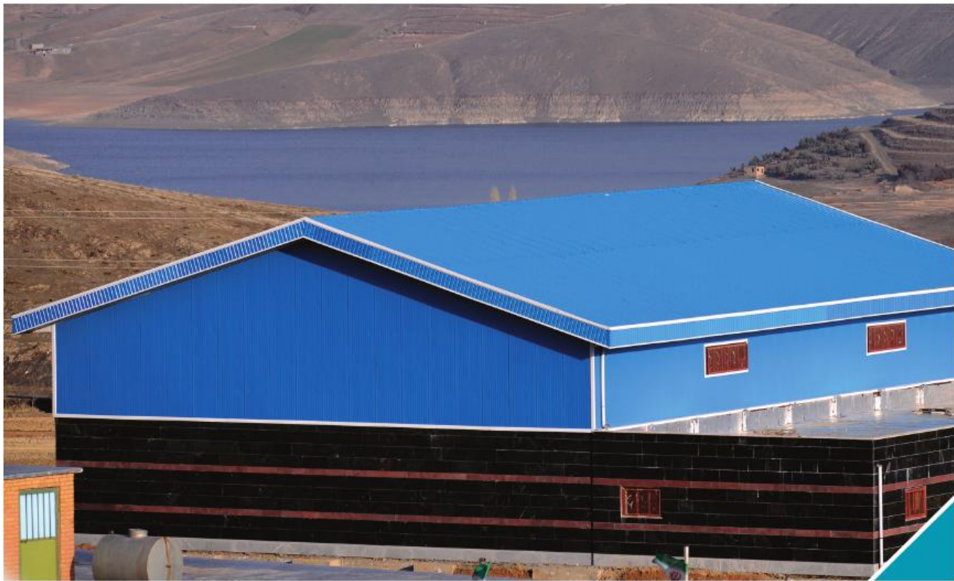
Roof of dairy center in Cremona
