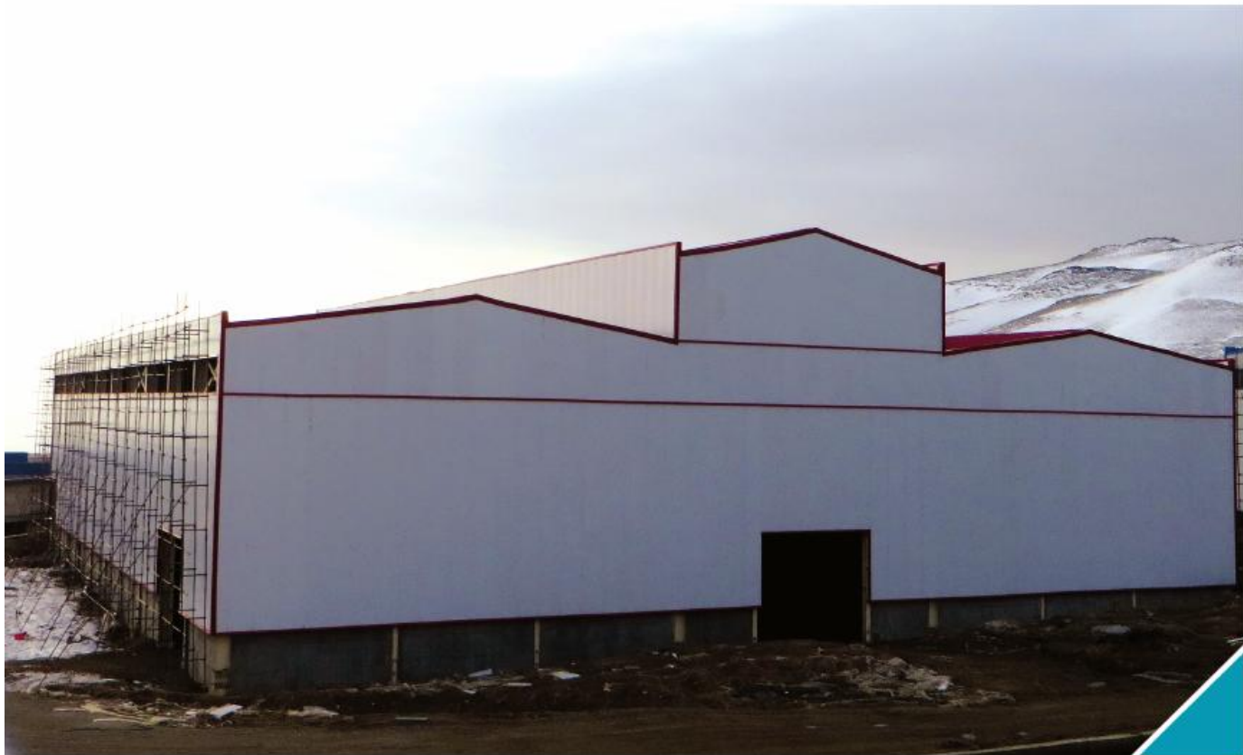
Roof of dairy center in Cremona
