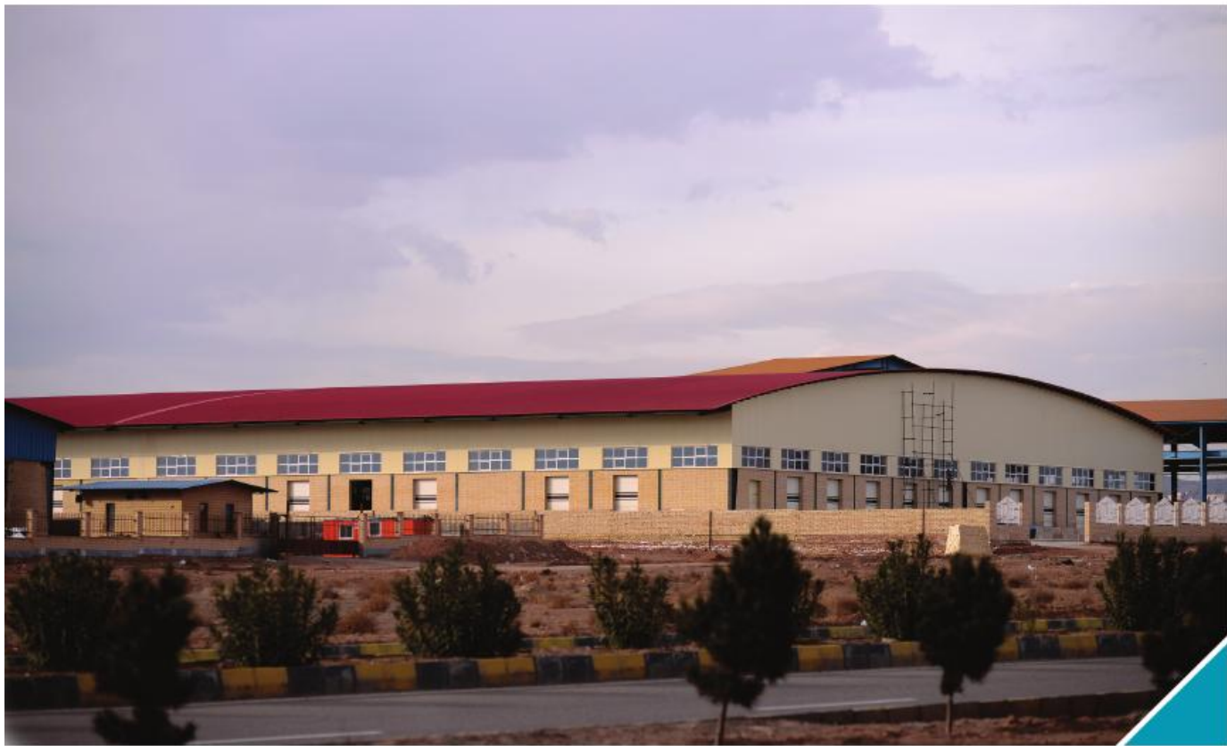
Roof of dairy center in Cremona
