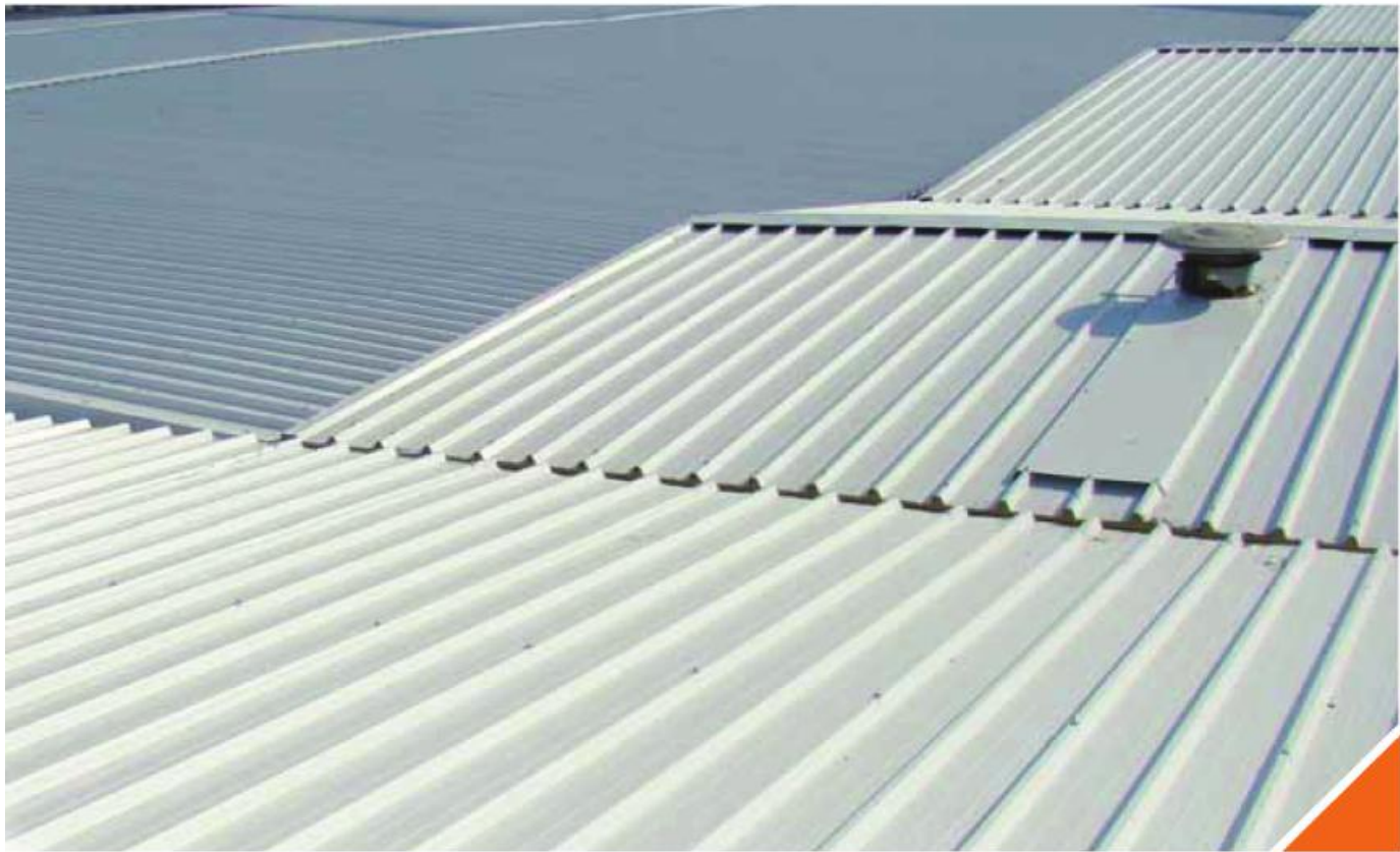
Roof of dairy center in Cremona
